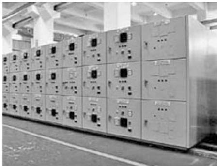
**FIGURE 7.1** Medium-voltage switchgear
