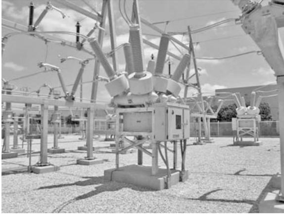
**FIGURE 7.8** SF<sub>6</sub> gas circuit breakers
