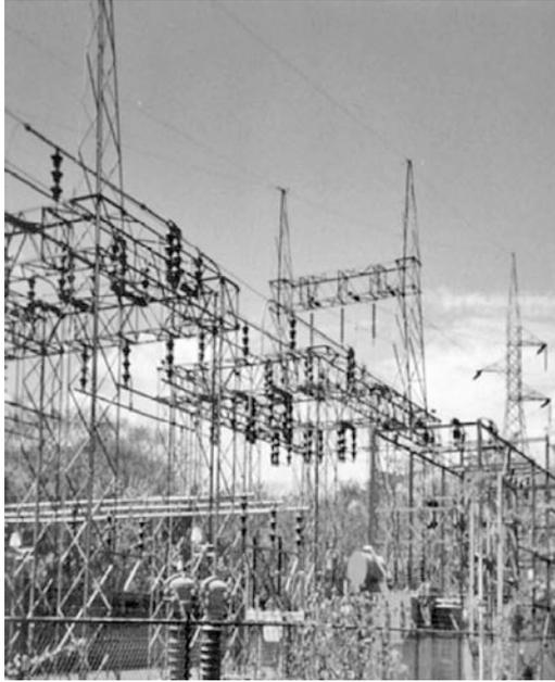
**FIGURE 12.16** Switchyard protected by overhead shield wires
