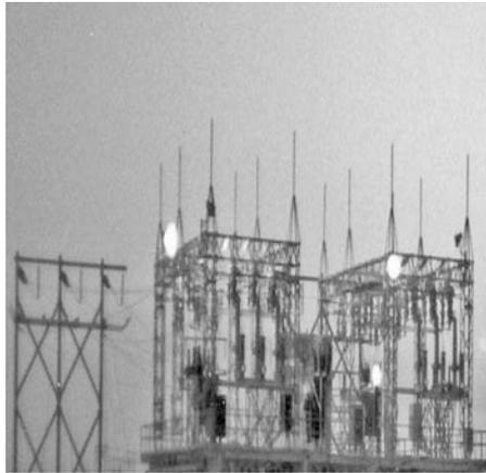
**FIGURE 12.17** Switchyard protected by masts
