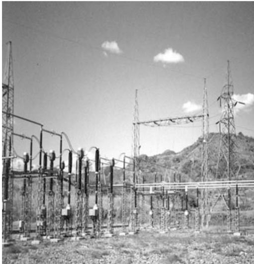
**FIGURE 12.14** Switchyard using rigid bus-work
